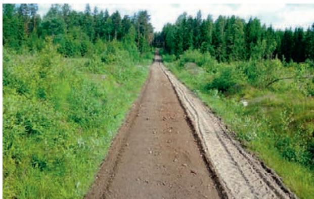
Vägen under bearbetning
